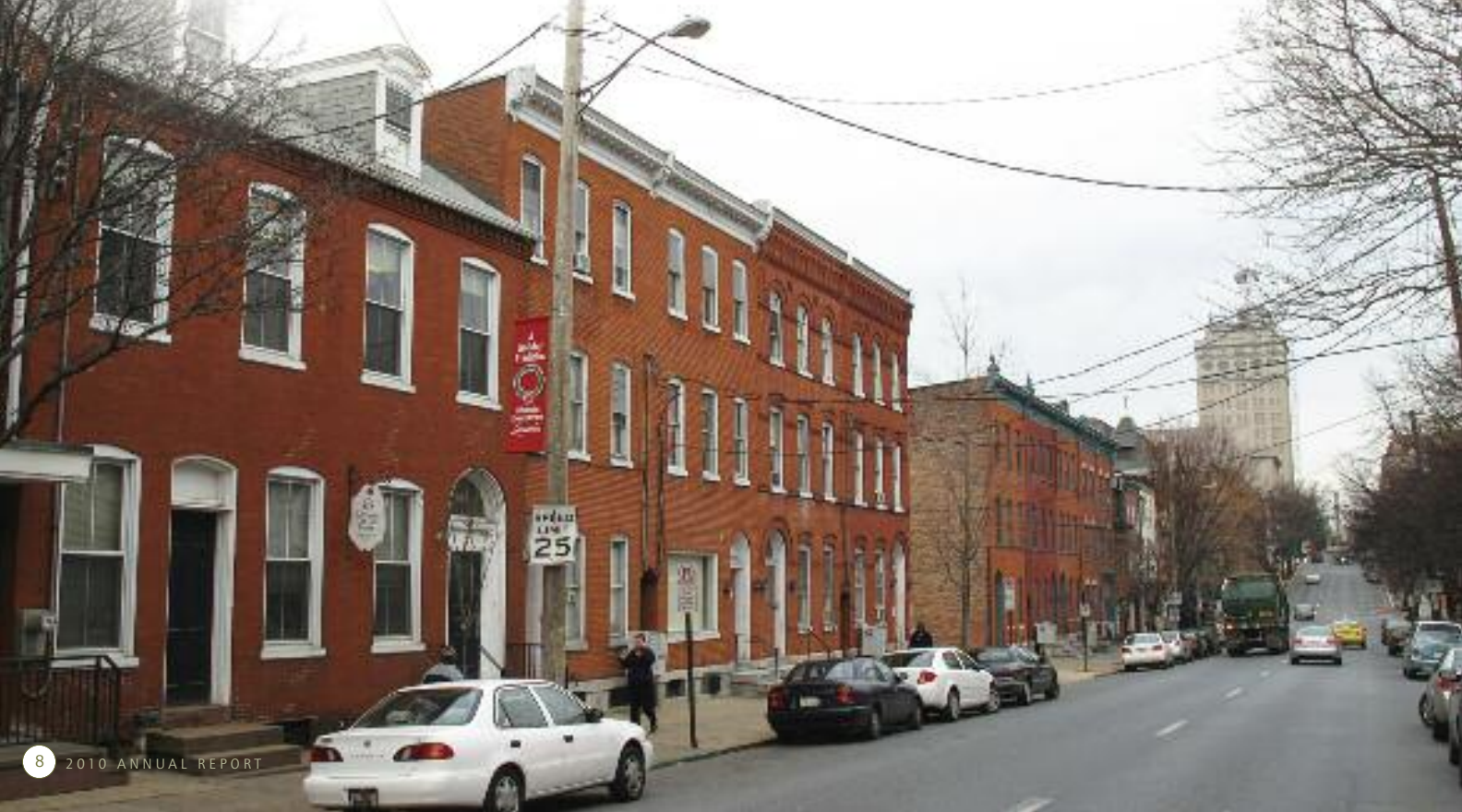
South Square will revitalize the 100 block of South Queen Street
