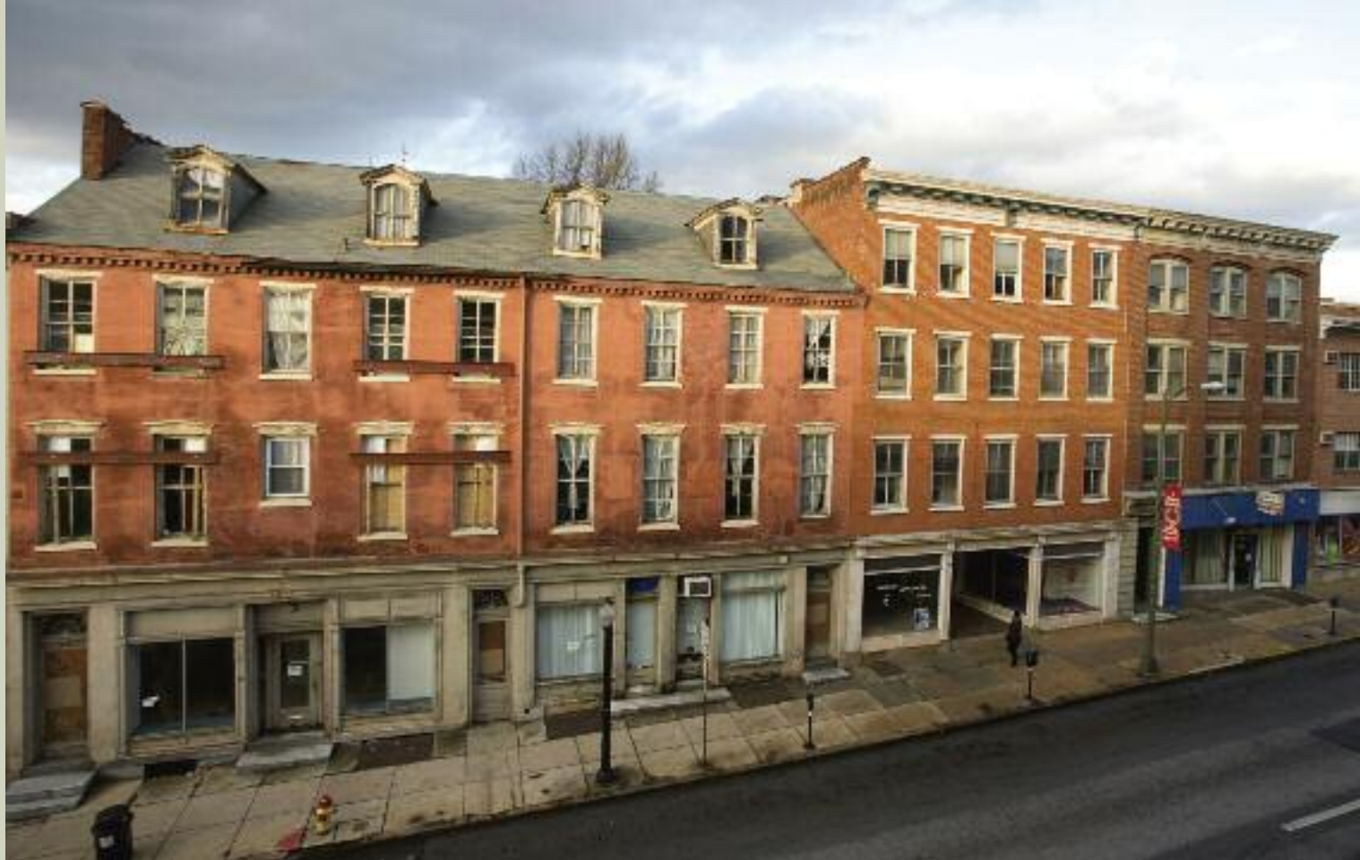
In the $8.5 million redevelopment of the first two blocks of East King Street in Lancaster City, the Historic East Side Suites project will feature both retail and residential properties.
